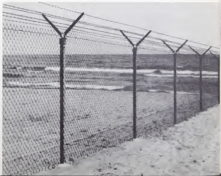
Here is a beach fence that really keeps a private beach private, yet it scarcely obstructs the view at all. The strands of barbed wire laid along the V-shaped arms are a sure discouragement to would-be trespassers. For a further description of this fence see page 21.
